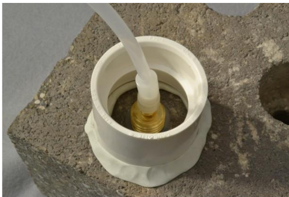
Figure 9. Water dam used for leak detection
